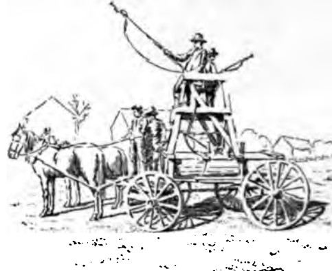
2378. Orchard pump with conical tower rig.
